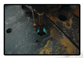
A stud welder gun provides a quick and strong method for applying the threaded studs to the steel floor through the counterbored holes.
